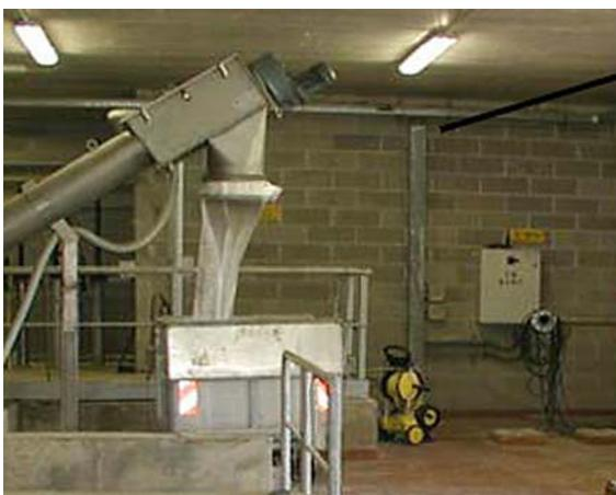
EMD Drum Screen fitted with screenings bagging system discharging to a container
